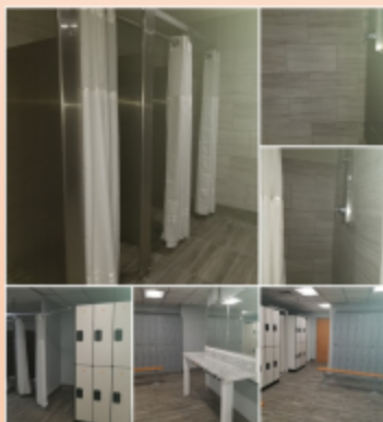
GIRL'S NEWLY RENOVATED LOCKER ROOM!
